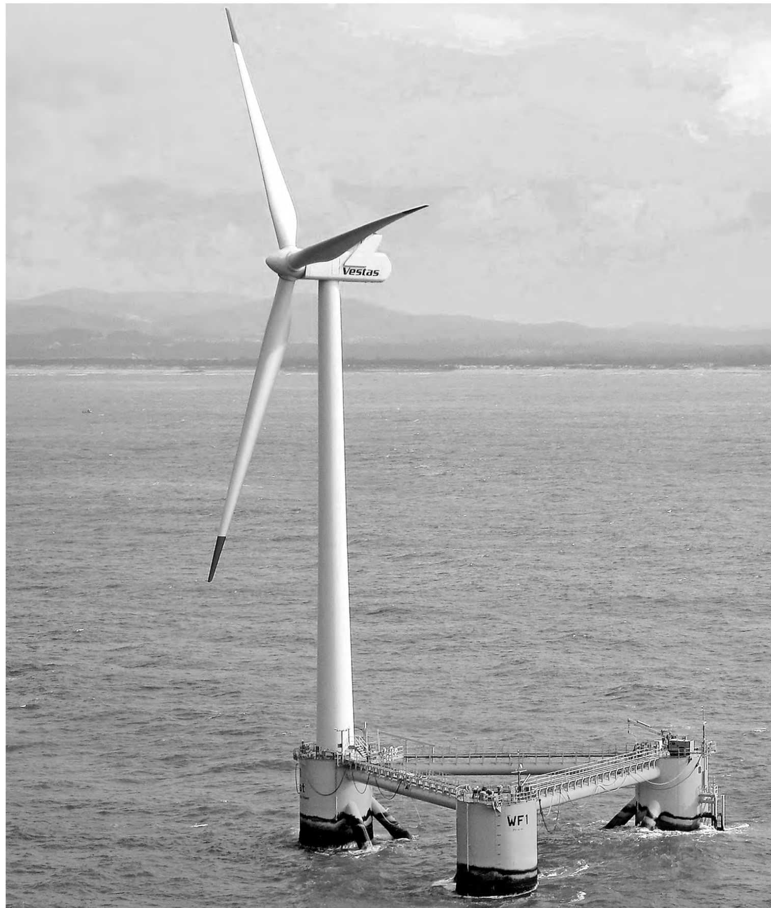
Wind instruments: semi-submersible platforms have been trialled off Norway and Portugal – Marc Preel / AFP / Getty Images
