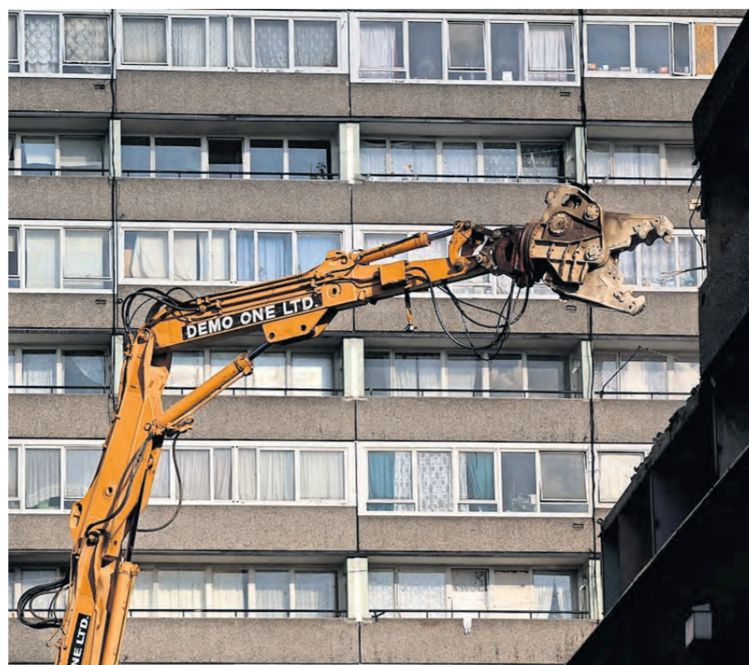
Painful: activists argue that demolition amounts to social cleansing — Oil Scarriff/Getty
