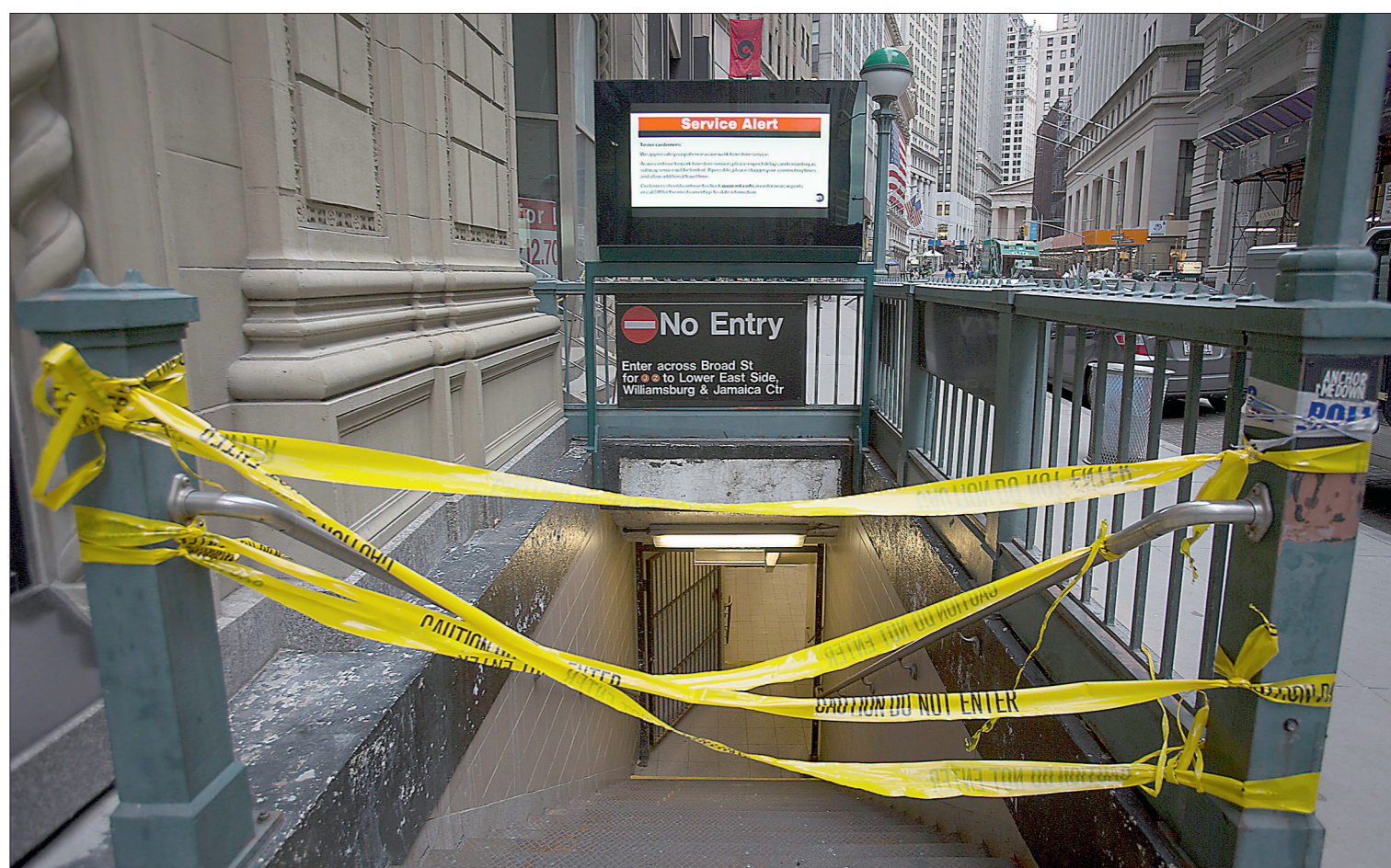
Storm damage: the NY metro was closed down after Superstorm Sandy struck
