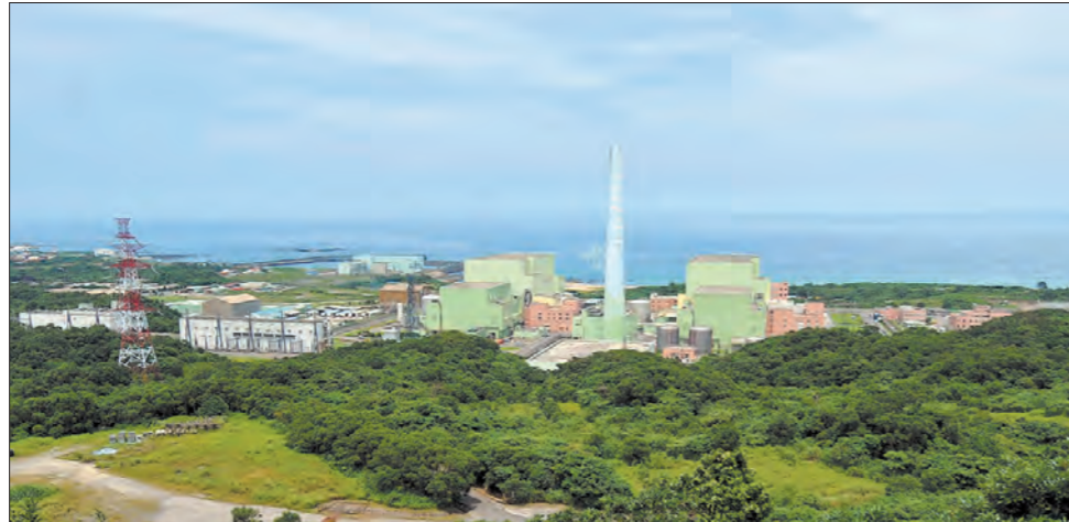
Allaying fears: Taiwan's fourth nuclear power plant in the northern Gongliao district
