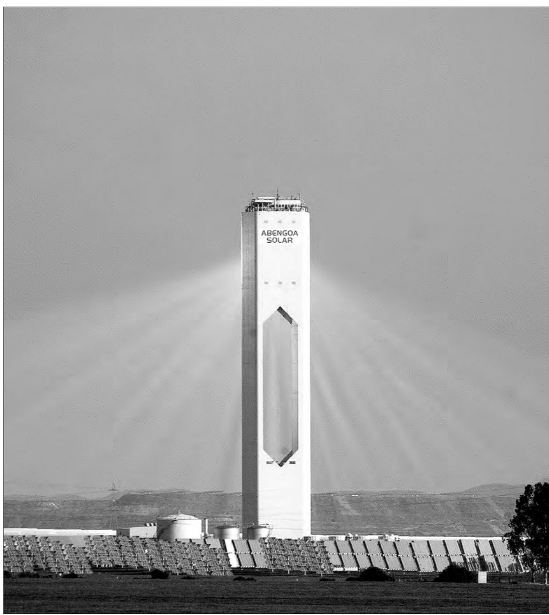
Power play: using sunlight to generate electricity in Sanlúcar La Mayor, Spain
