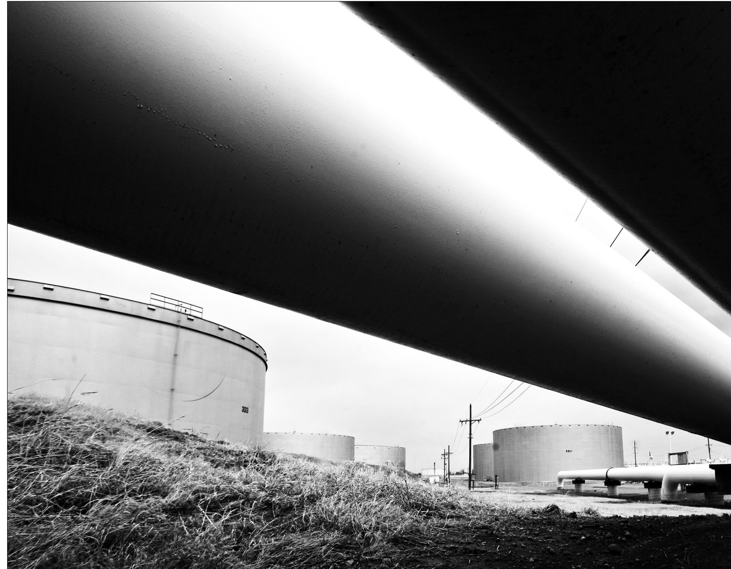
Crude estimates: one company sends a helicopter above the Cushing complex to gauge inventory levels, another uses a satellite Bloomberg
