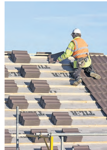
On out on the tiles: roofers at work
