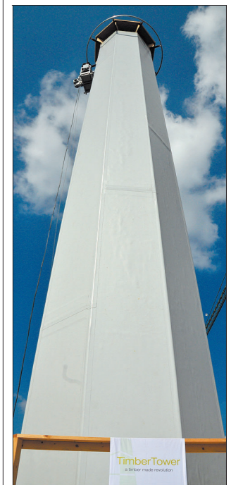
Spruced up: TimberTower's wooden turbine tower
