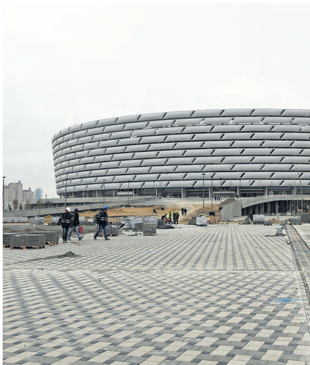
Finishing line: the vast national stadium in Baku nears completion
