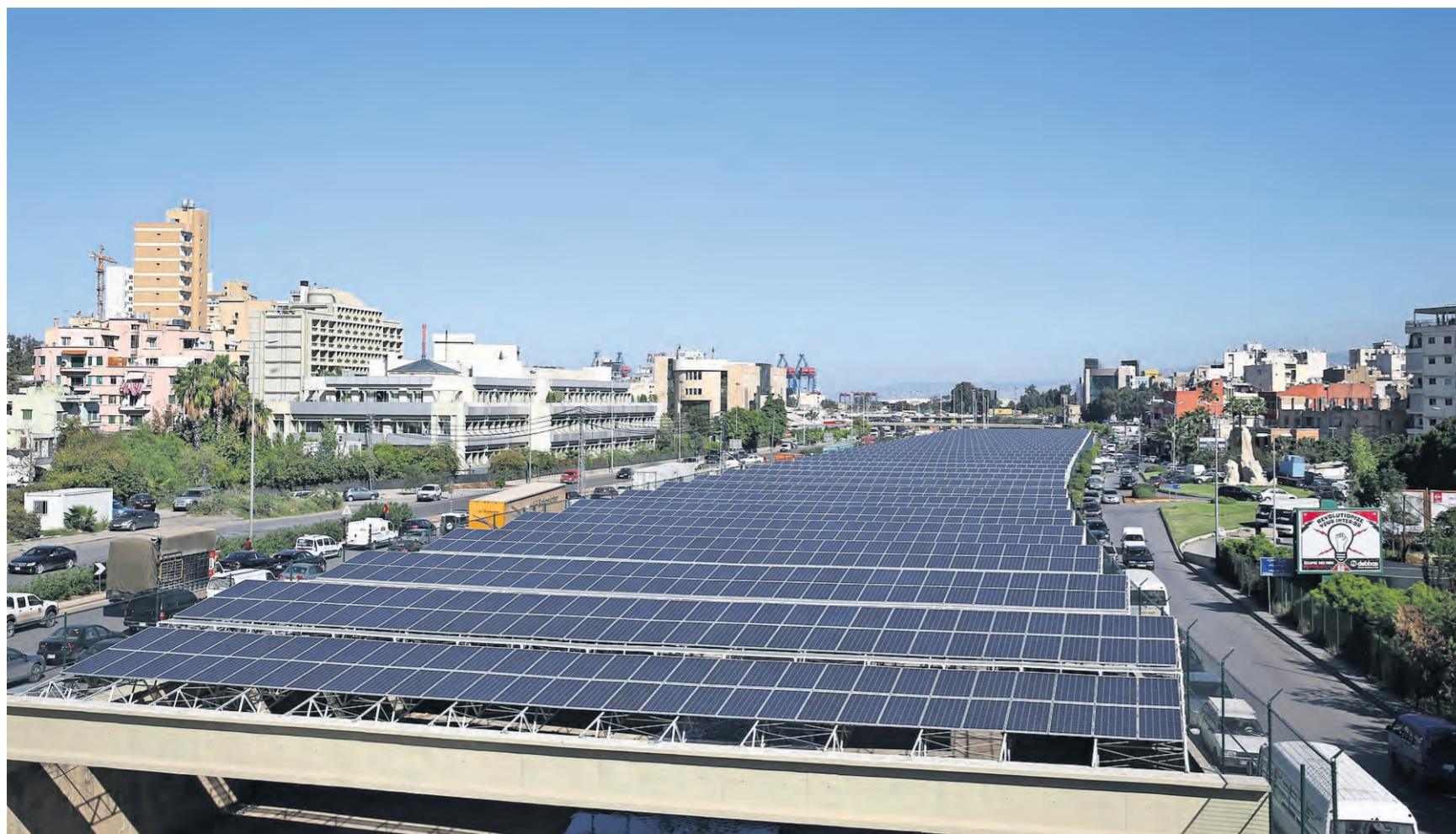
Photovoltaic progress: a view of the Beirut River Solar Snake, a 30m wide installation of PV panels over a river bed in the Lebanese capital — Joseph Eid/AFP/Getty Images
