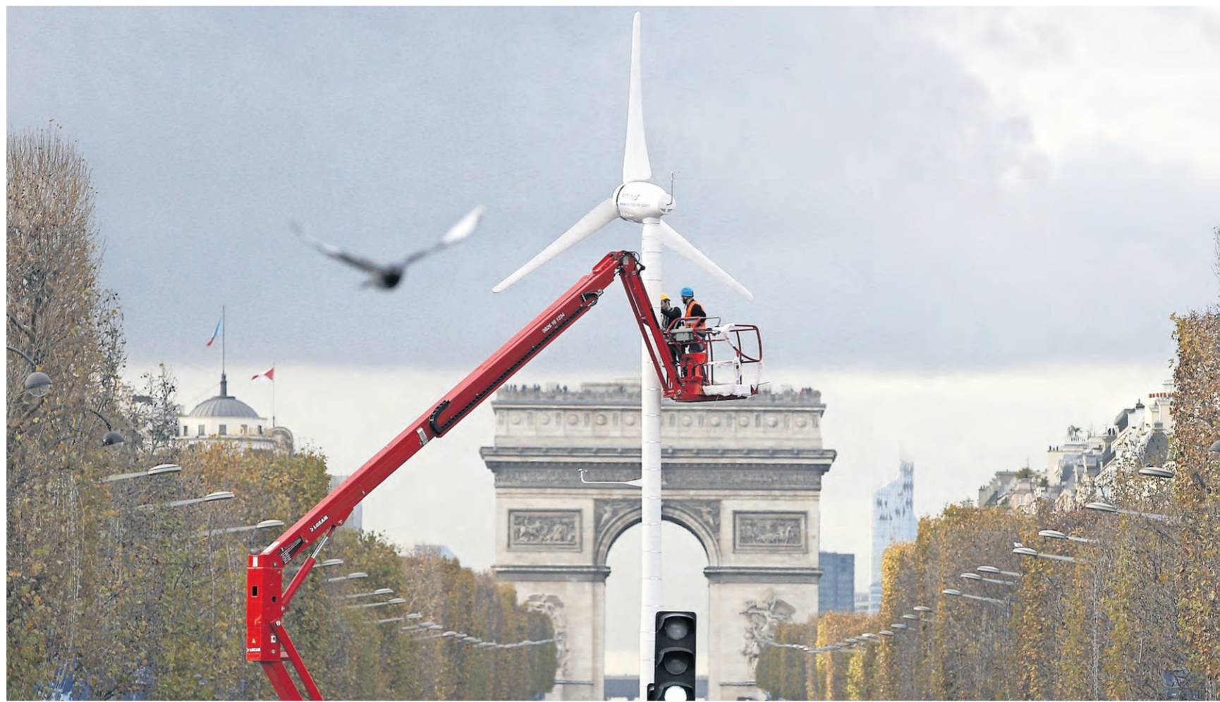
Installing for time: workers position a wind turbine on the Champs-Élysées before the Paris climate talks aimed at curbing global warming — Patrick Kovarik/AP/Getty Images
