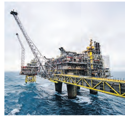
Oseberg A gas platform
