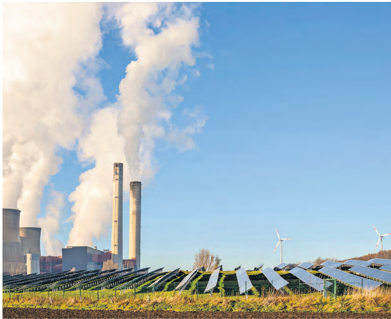
Out with the old, in with the new: power plant, solar panels and wind turbines sit together in Germany — Alamy
