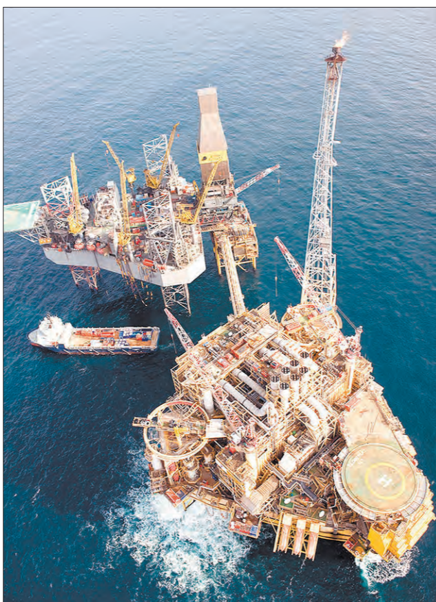
Shutdown: the Elgin platform, right, before the blowout
