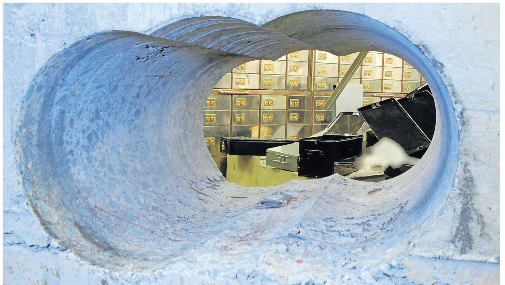
Thieves drilled through a thick concrete wall to access a vault in Hatton Garden, London Getty
