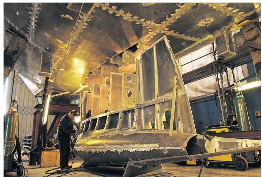
Teamwork: Pendennis has more than 360 skilled tradespeople at its yard
