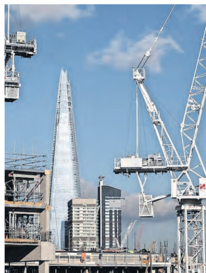
Construction near London's Shard
