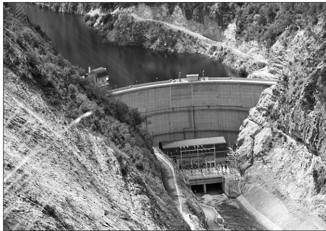
Overhaul: Sveta Petka, Elem's automated hydropower plant
